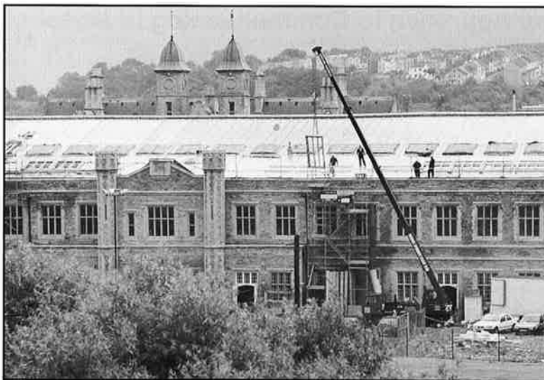
'Restoration in progress, Passenger Shed roof bay being replaced, 1997'
