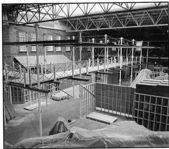
'The courtyard showing the walkway under construction'
