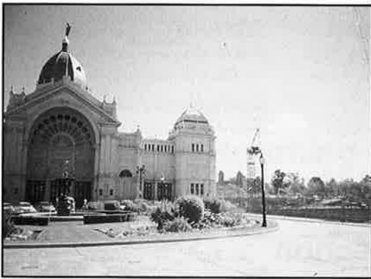
Work begins on the new wing alongside the 1880 Royal Exhibition building - the new home of the Museum of Victoria at Carlton Gardens, Melbourne.
