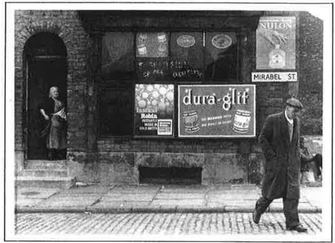
Photograph © Shirley Baker, Mirabel Street 1965
