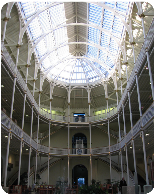
Cast iron construction in the Royal Scottish Museum, Edinburgh.
